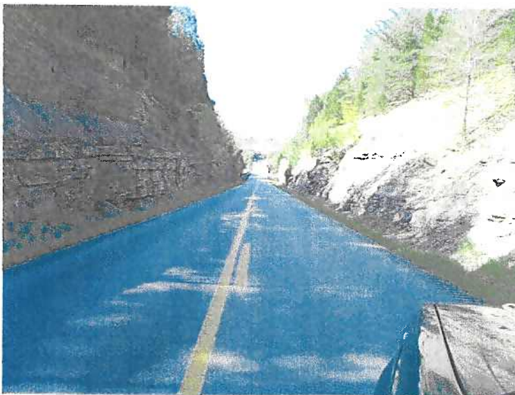
KY 88 typical cut on hill
